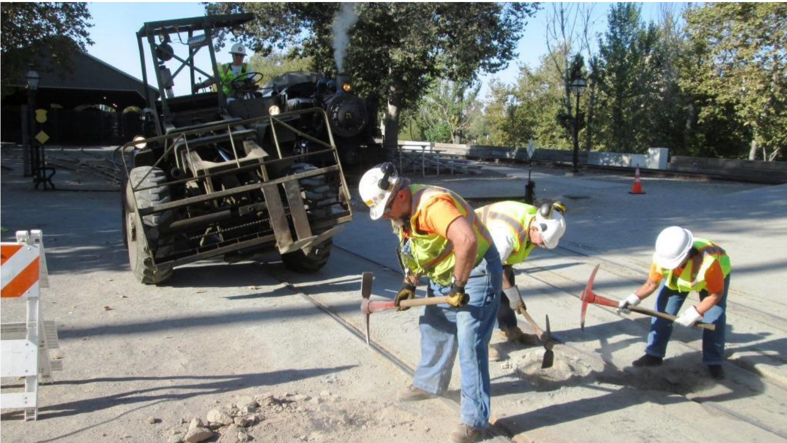
Mike F., Clem, and Pam chip away at the dirt near the edge of the concrete as Mike H. "break-dances" on Big Green
