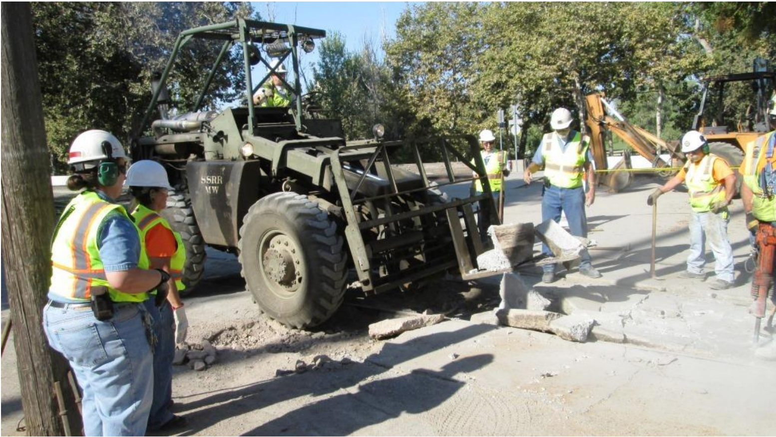
More concrete demolition by Big Green
