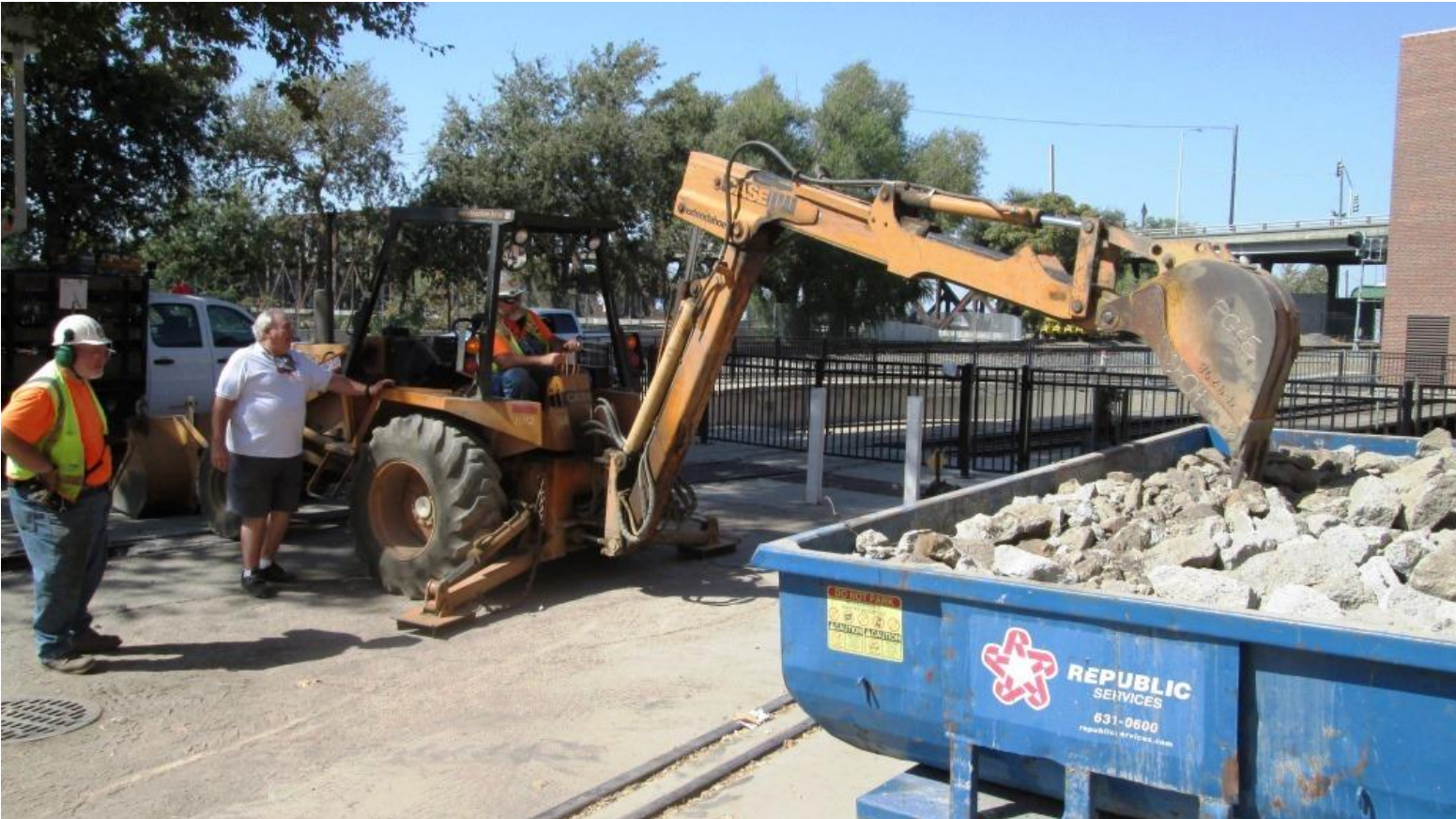
Harry Voss stops by to watch Mike F. on the back-hoe even-out the concrete chunks in the dumpster
