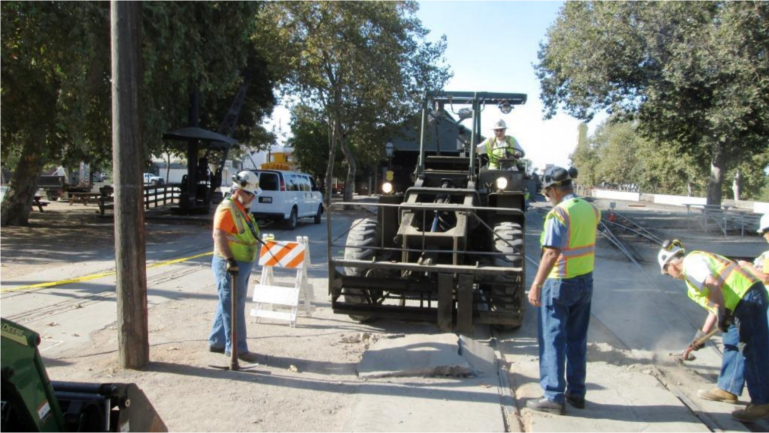
Mike H. gets the forks of Big Green under the concrete and lifts it out
