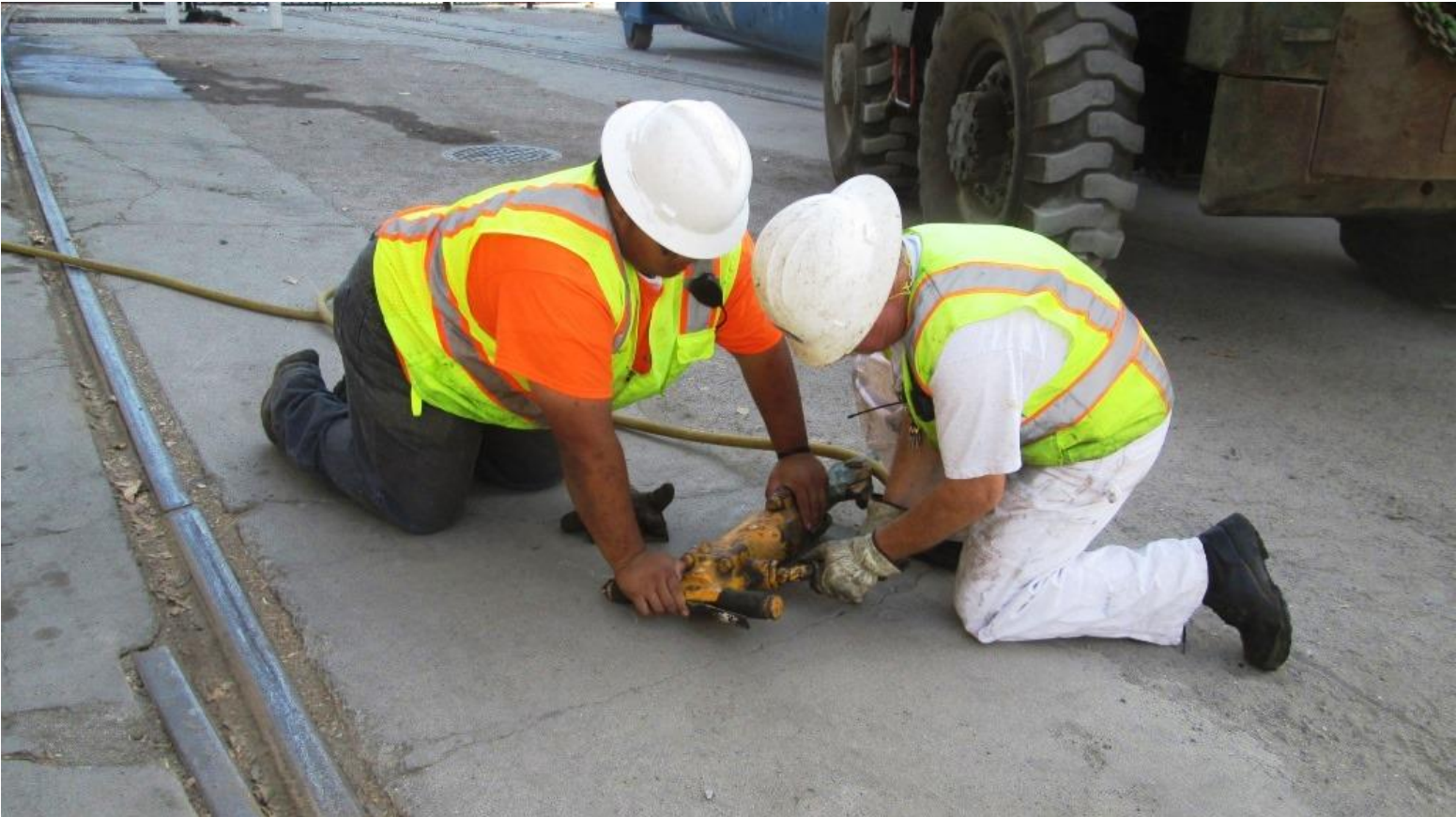
Anthony and Mike H. attach the air-hose to the jack-hammer
