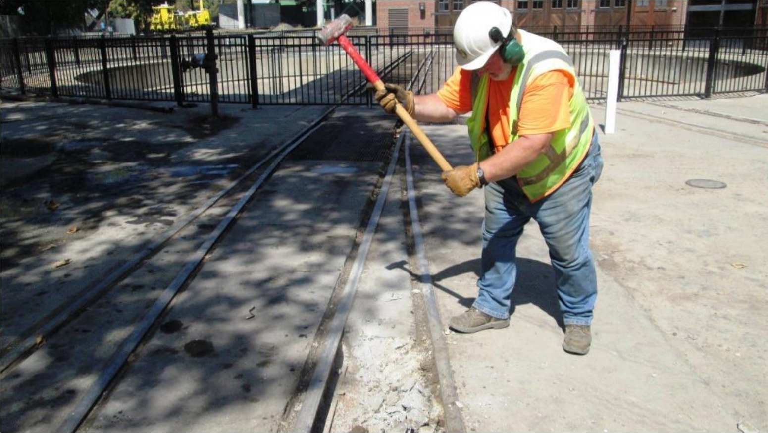
Frank breaks-up the concrete going into the wedge of the switch
