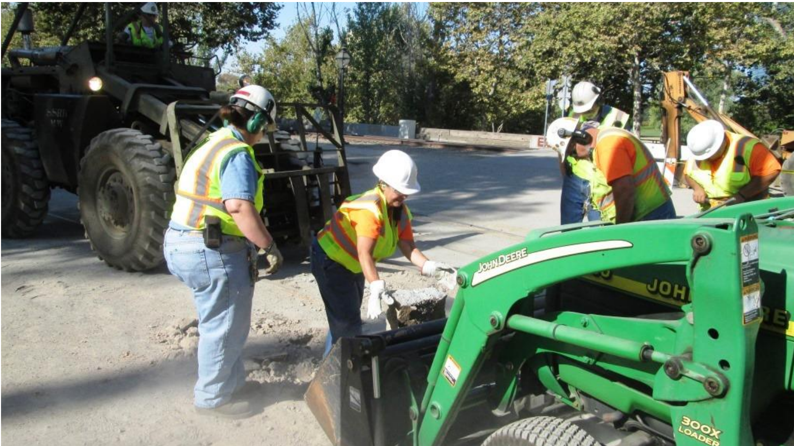
Heather and Pam move more concrete into the bucket
