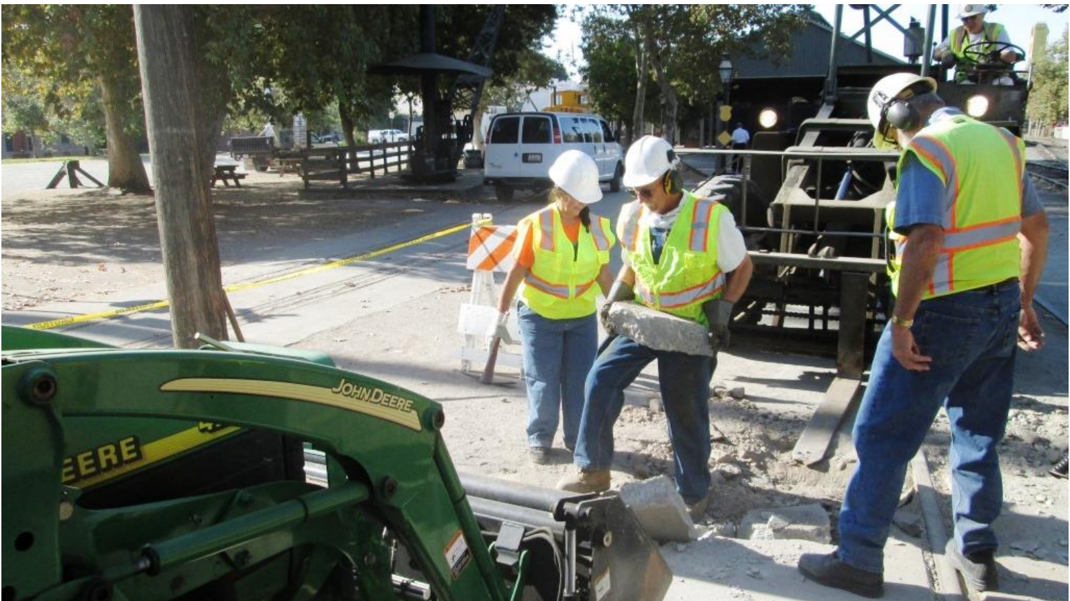
Clem and Pam move concrete blocks as part of the MOW Team "chain-gang"
