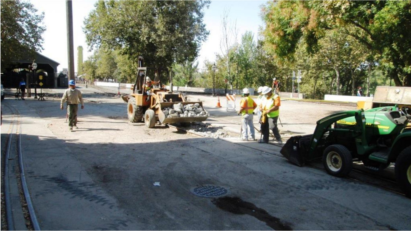
Mike F. on the back-hoe takes a bucket full of rubble to the dumpster
