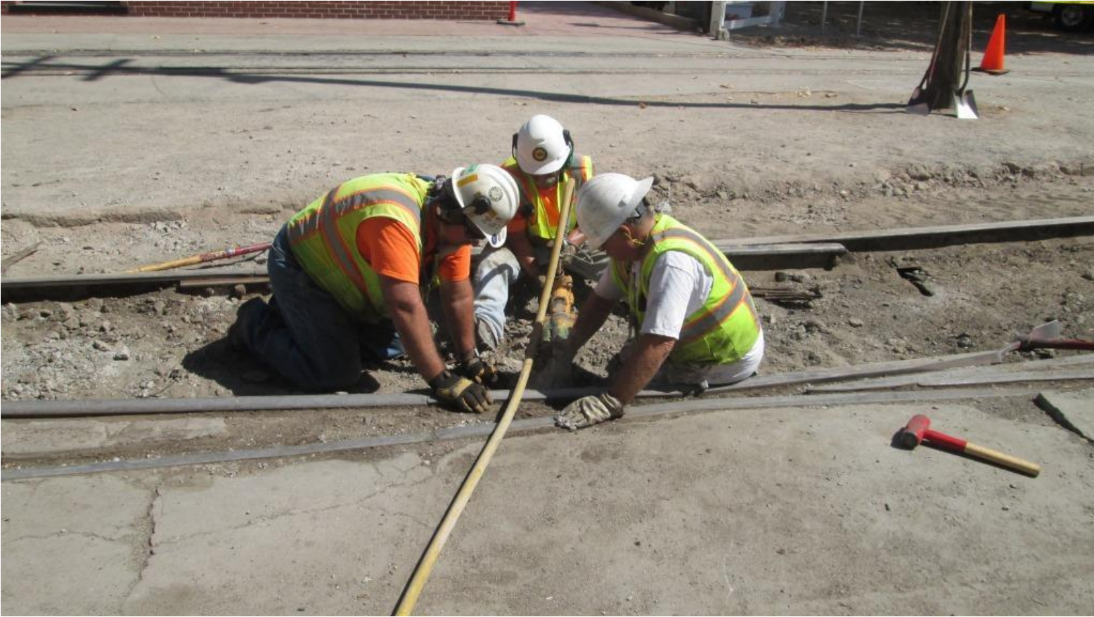
Jack-hammering out concrete stuck between bolts is proving more difficult than initially believed...
