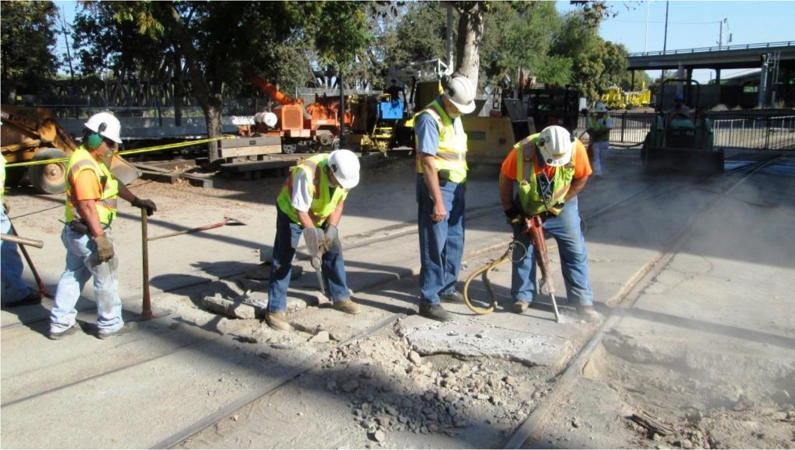
Joe and Clem pick away at the edges concrete with mattocks tools while Alan guides Mike F.'s efforts on the jack-hammer
