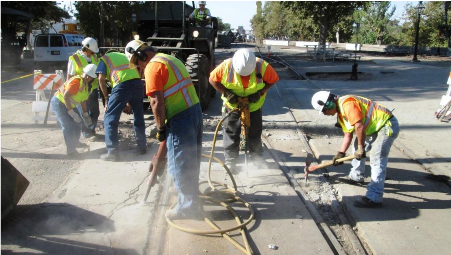
Mike F. and Anthony tag-team the concrete
