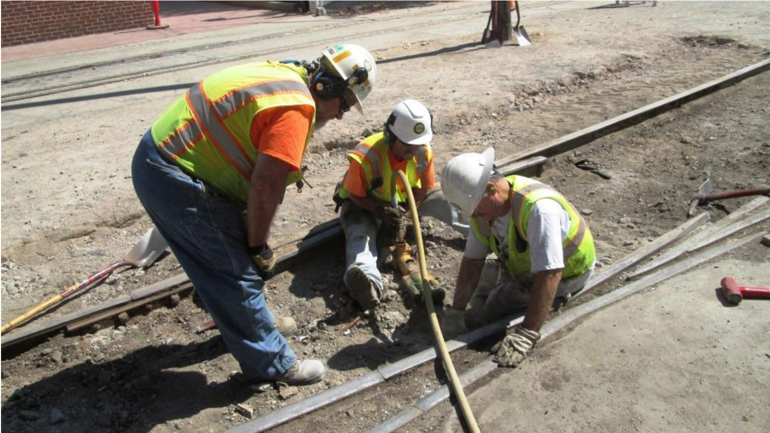
Mike F., Joe, and Mike H. set up for horizontal jack-hammering
