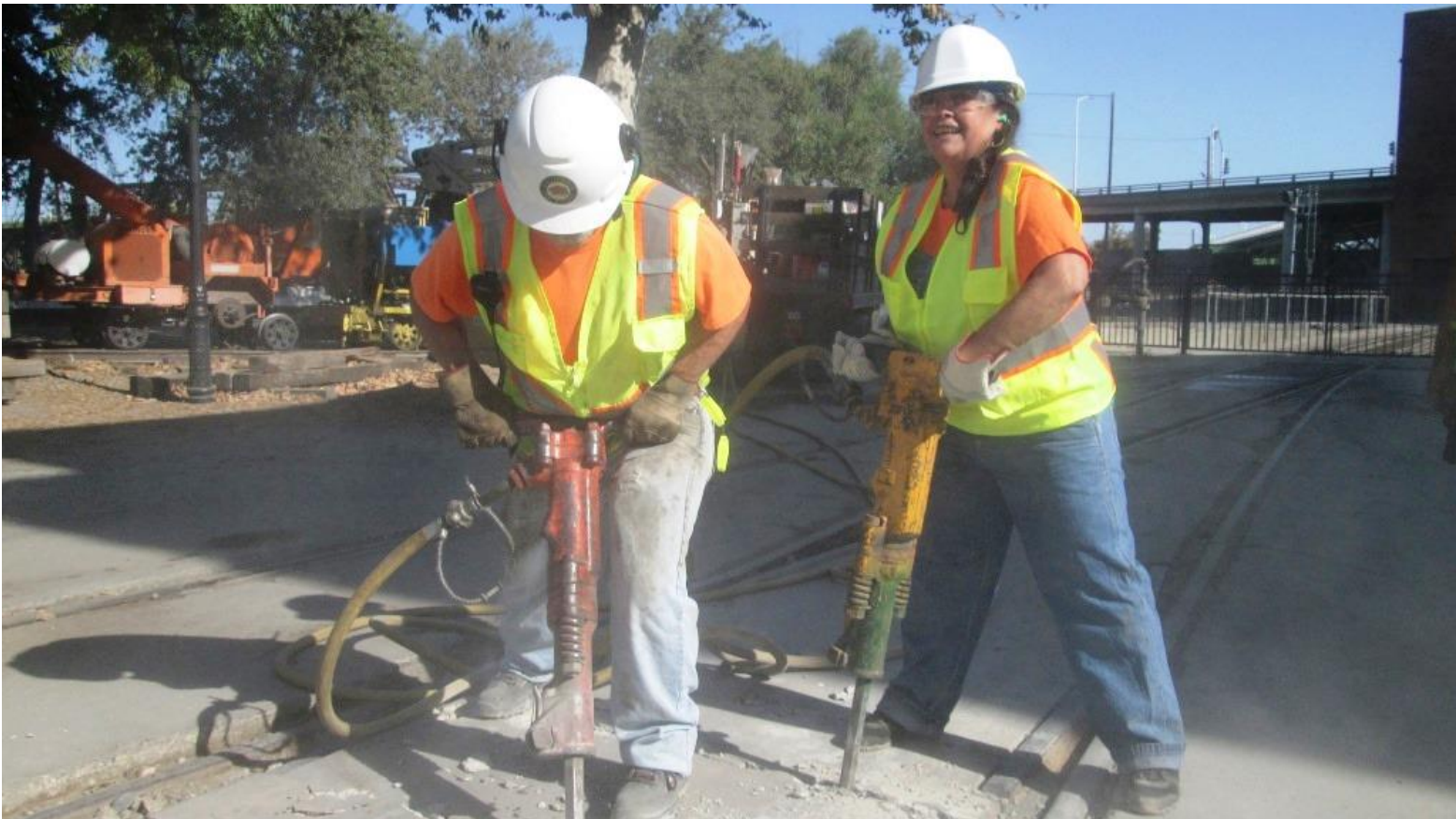
There's no doubt that Pam thinks that breaking out concrete with the jack-hammer is fun!
