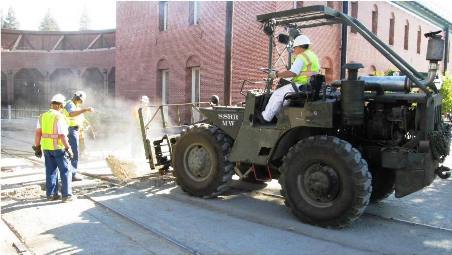
Mike H. lifts-out more concrete with Big Green
